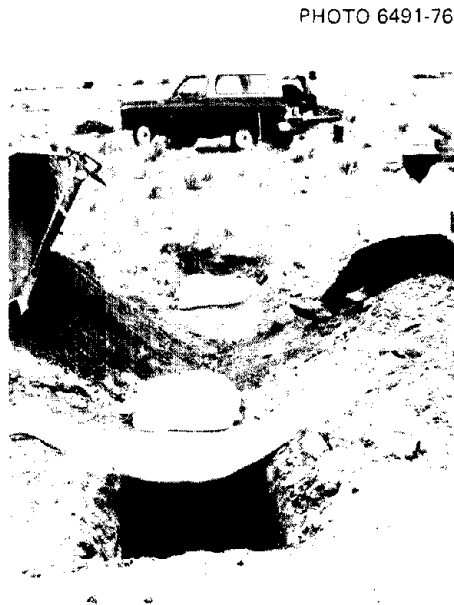
Fig. 12.3. Dumping earth on side of rug before mounding earth 4 ft deep along centerline. An earth-filled bed-sheet "roll" and a pillowcase "sandbag" retained earth at each entry, pictured prior to completion.
